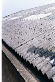
Asbestos roof
